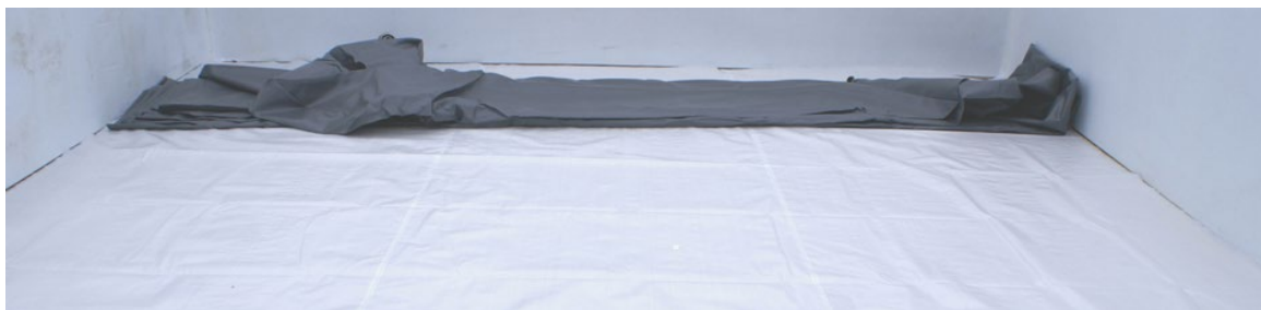
Figure 33 – Unfolding the liner
