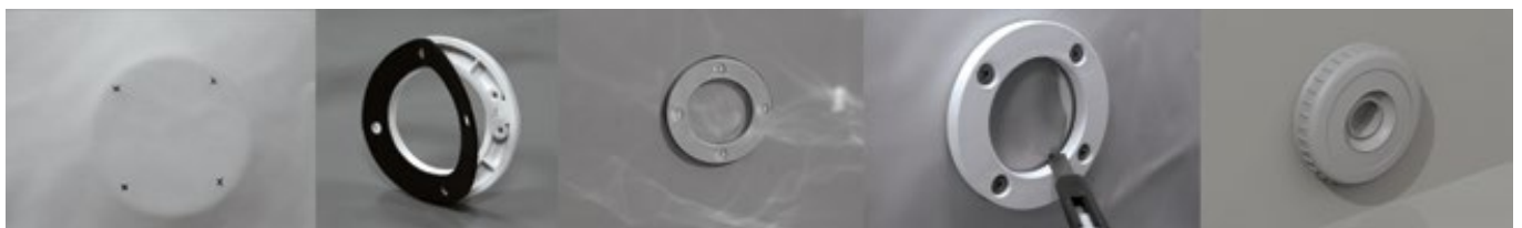
Figure 35 – Installing the return fitting flange
